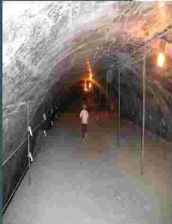
Top of tunnel passageway usually off limits to the public.
